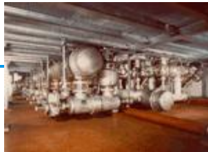
Gas-insulated switchgear
